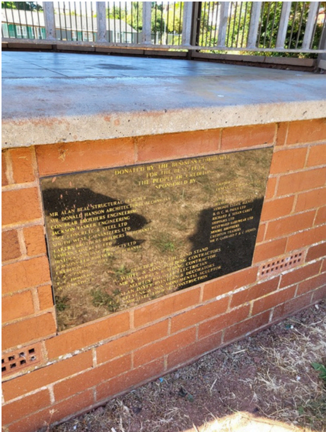
Image 5: Plaques in good condition
