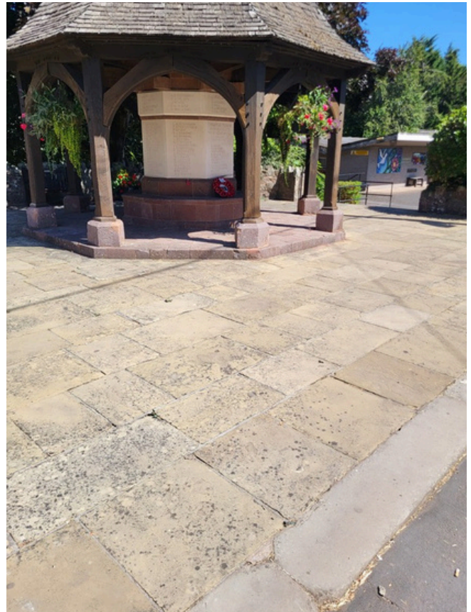
Image 2: External slabs are clean and weed-free
