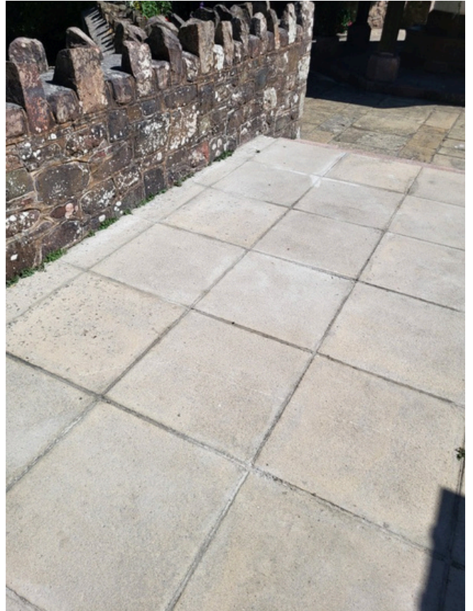
Image 6: Rear slabs in good condition - cleaned, weeded and repointed
