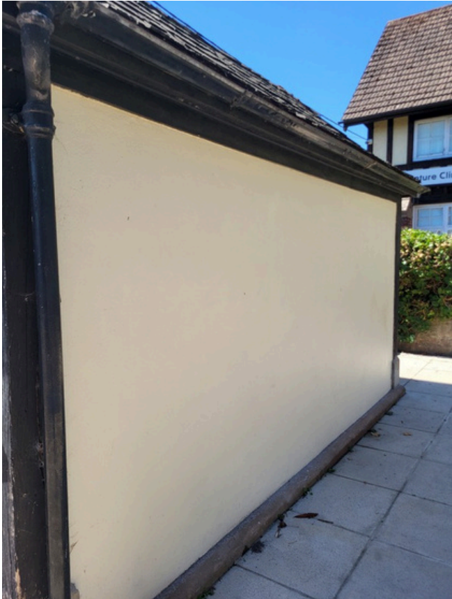
Image 5: Rear wall, clean and great condition
