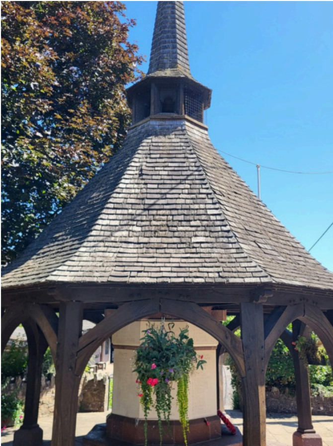
Image 10: West elevation - roof shingles in good condition
