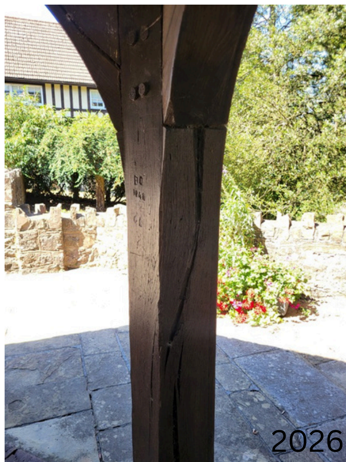
Image 7: Cracks to uprights. No change from previous inspection.
