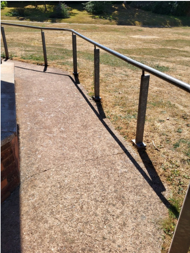
Image 9: Ramp is clean with no defects
