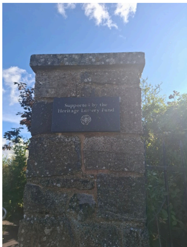
Image 11: External plaque in good condition
