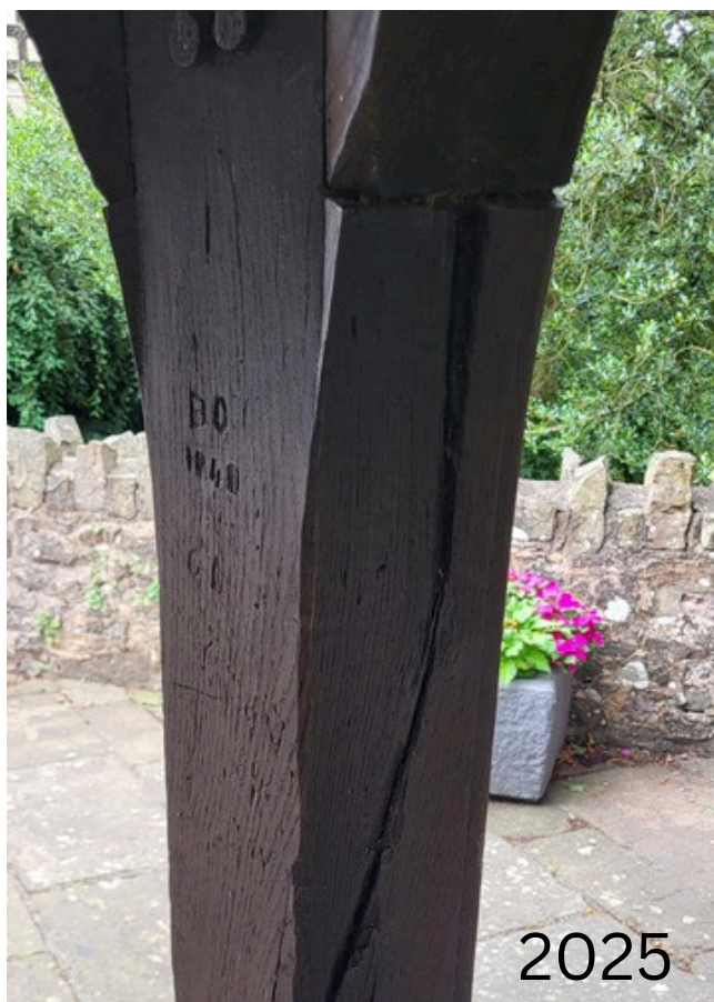
Image 7: Cracks to uprights. No change from previous inspection.
