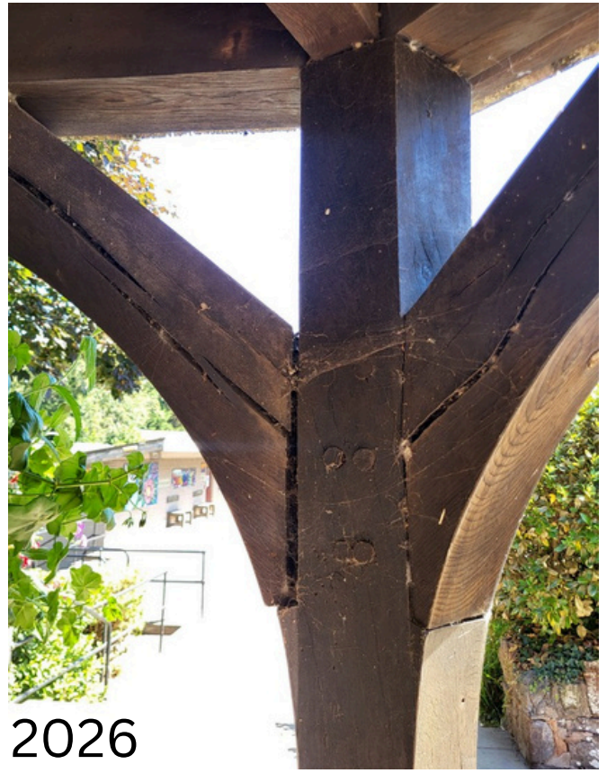
Image 5: Cracks to uprights. No change from previous inspection
