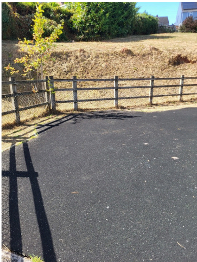
Image 3: Fencing in good condition
