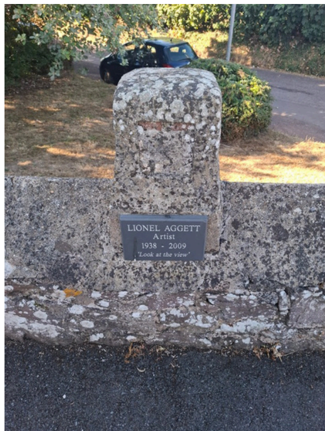
Image 10: Internal plaques in good condition
