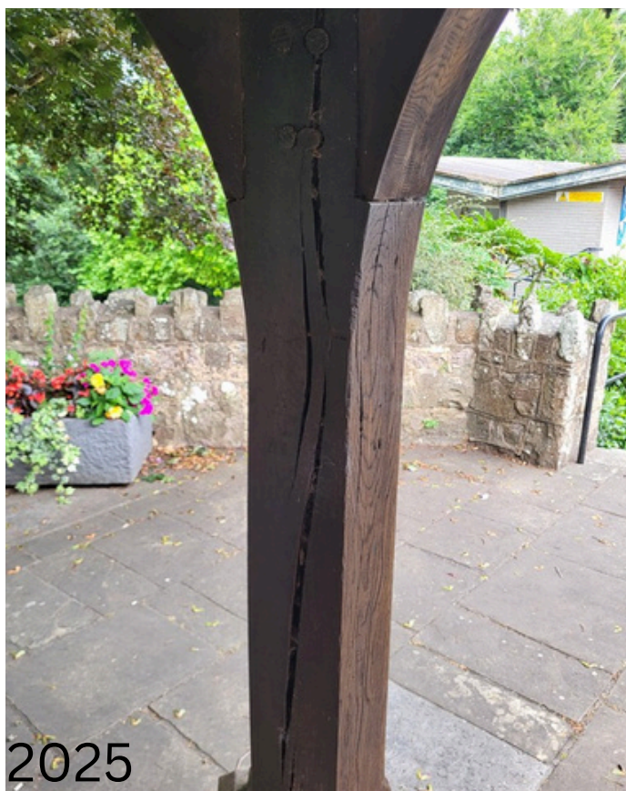
Image 6: Cracks to uprights. No change from previous inspection
