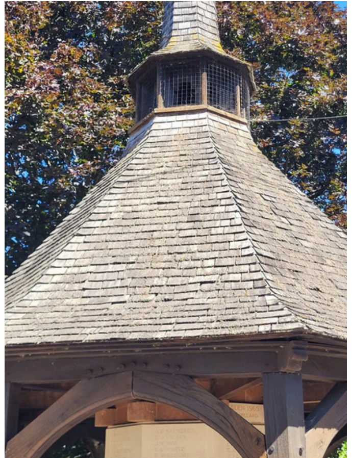
Image 11: Front elevation - roof shingles in good condition
