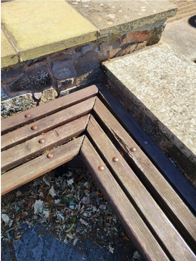
Image 9: Small section of wood on bench that has come away, no action required.
