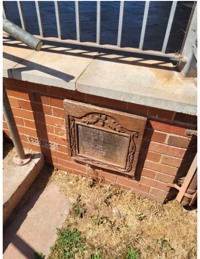
Image 6: Plaques in good condition
