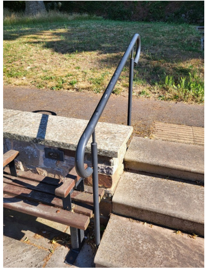
Image 6: Clean handrails, small amount of flaking paint
