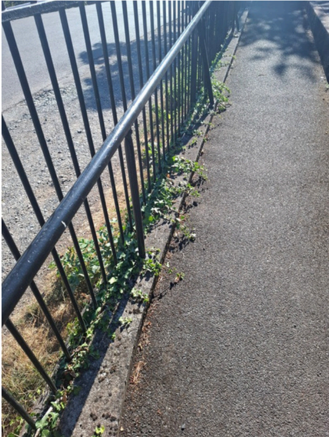
Image 1: Railings in good condition
