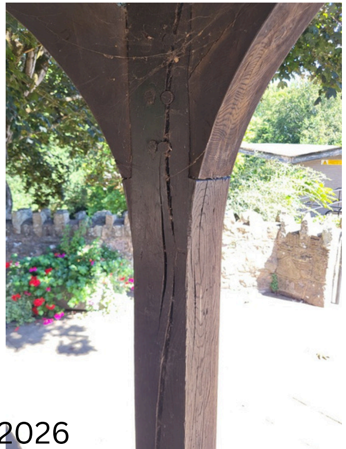
Image 6: Cracks to uprights. No change from previous inspection
