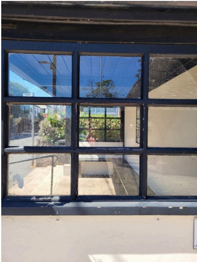
Image 4: Slight peeling to paintwork but overall good condition
