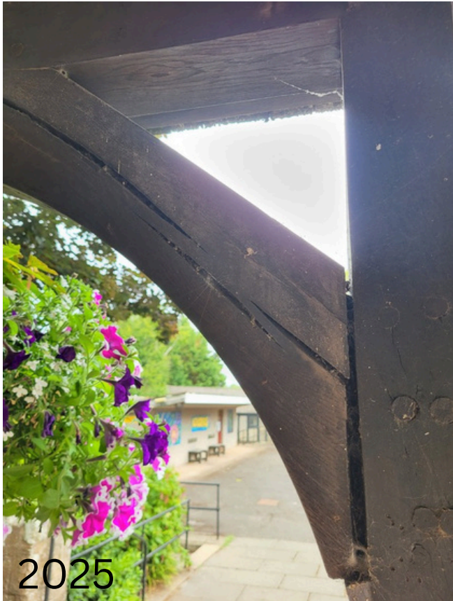
Image 5: Cracks to uprights. No change from previous inspection
