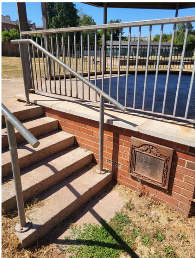
Image 7: Steps are clear with no defects
