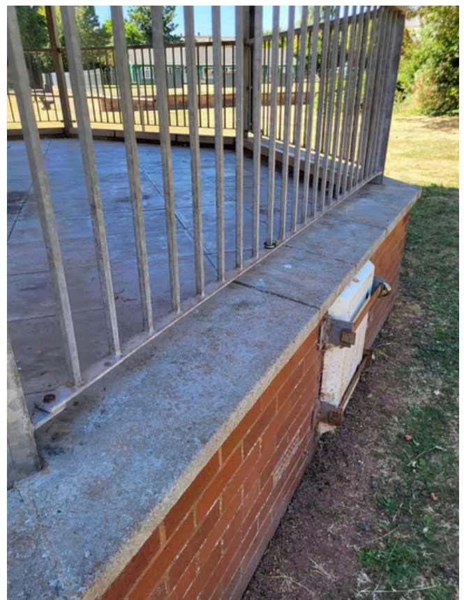
Image 8: Wall and pointing in good clean condition
