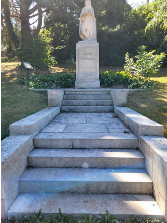
Image 1: Steps and slabs clean condition
