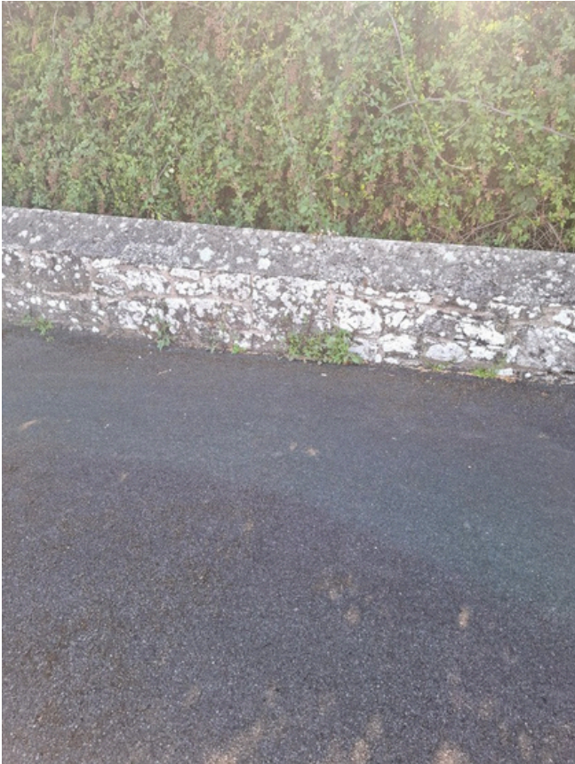
Image 5: Tarmac in good condition
