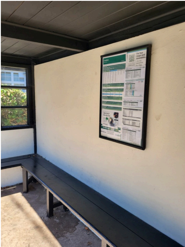
Image 1: Internal walls and benches
