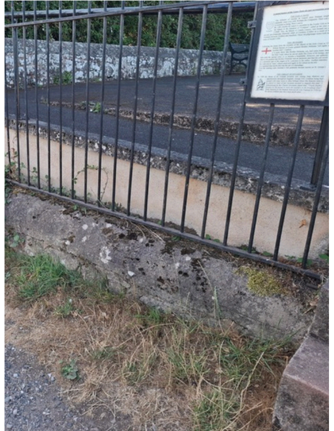
Image 2: Railings in good condition
